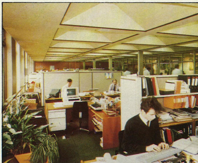
The office space, showing ceiling coffers incorporating lighting.
